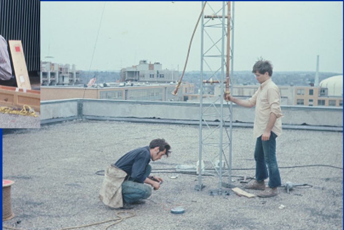
Ted Dudziak (right) with a tower rigging contractor.
